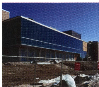
The new exterior features large windows near the auditorium
